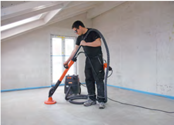
Grinding screeds
