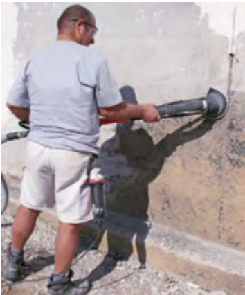
Grinding bitumen coating with PCD grinding disc
