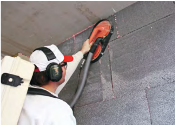
Grinding EIFS and ETICS boards
