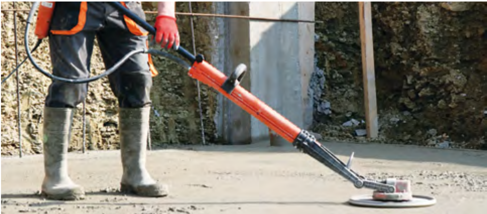
Levelling fresh concrete
