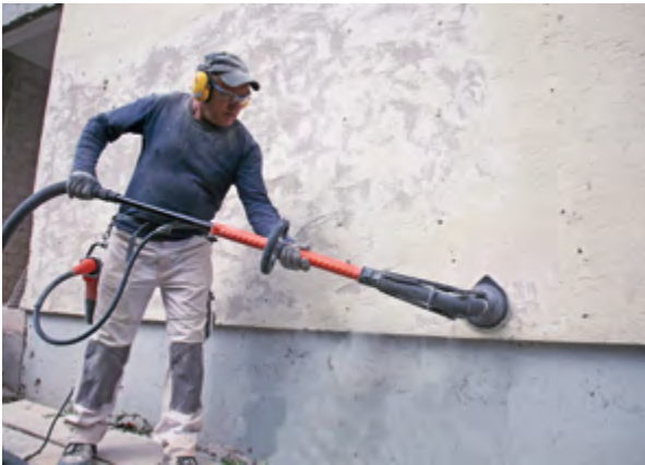
Removing old plaster and paints
