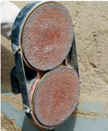
Removing old plasters
